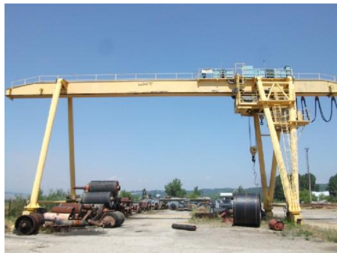
Figure 1. MPT 20/5 gantry crane
